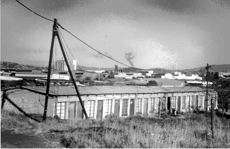
Figure 5. A row of concrete imijondolo in the informal settlement. Each umjondolo is rented for R60 a month. Isithebe Industrial Park is visible behind.
